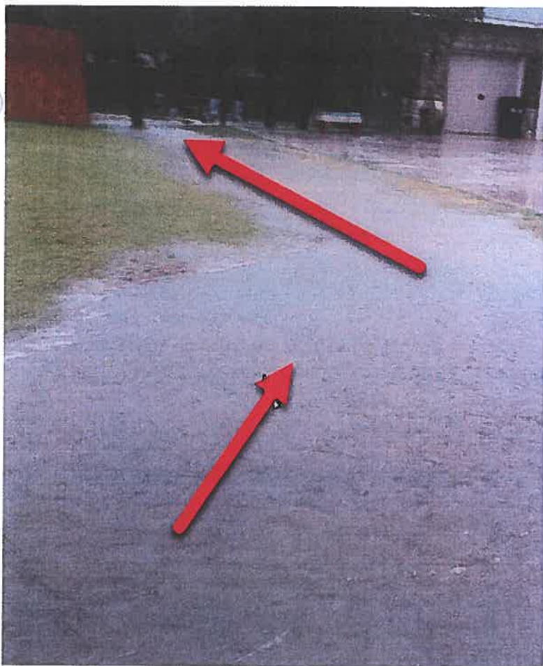
3rd photo, Backyard water flows from left to right towards their property.
